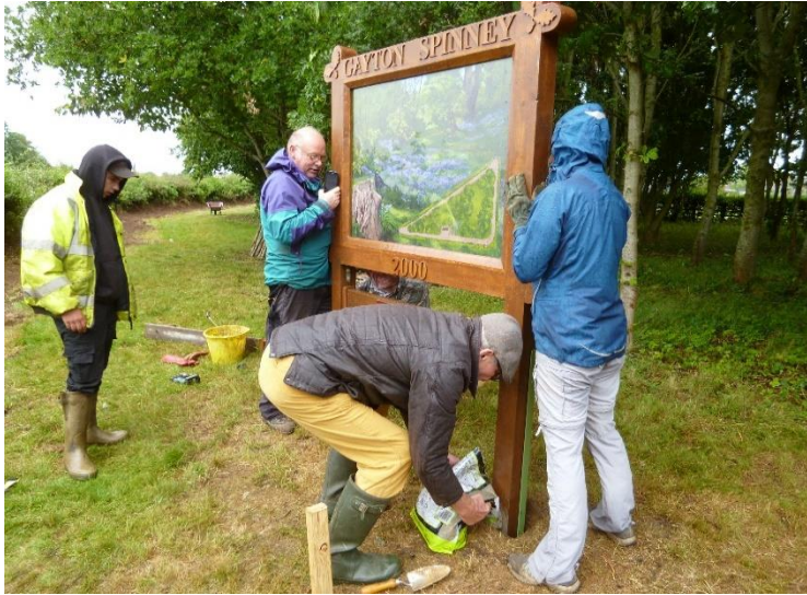
Filling the holes with concrete
