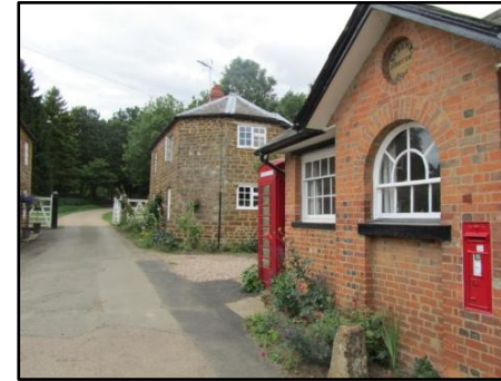
Walk 1: Hulcote, old school building.
